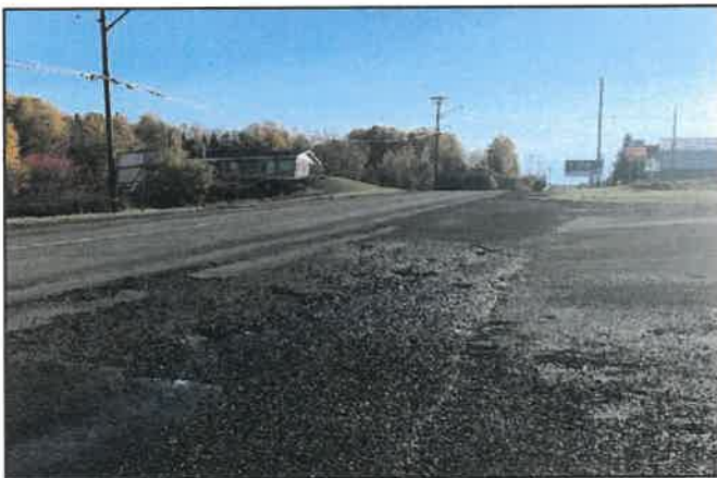
Figure A: east of the existing driveway access
